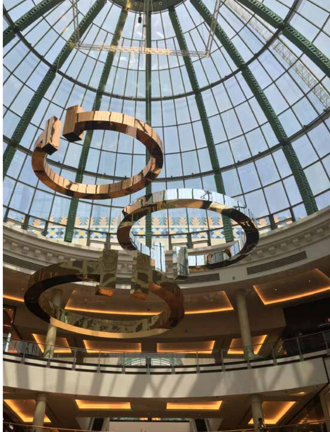
Aluminium Truss - Fountain Area - Mall of Emirates
