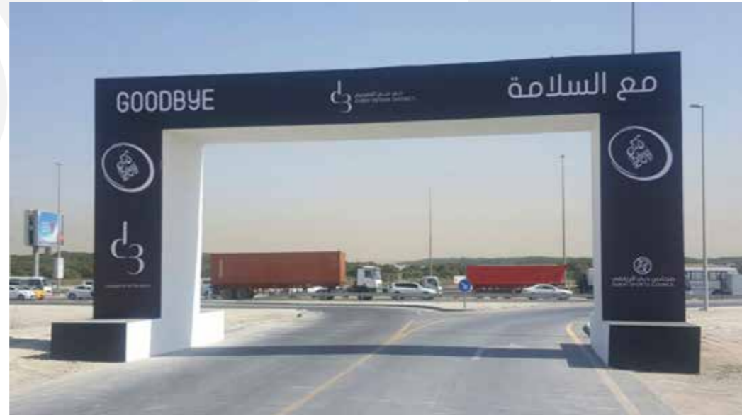
Wide Span Archway Structure - Buisness Bay D3
