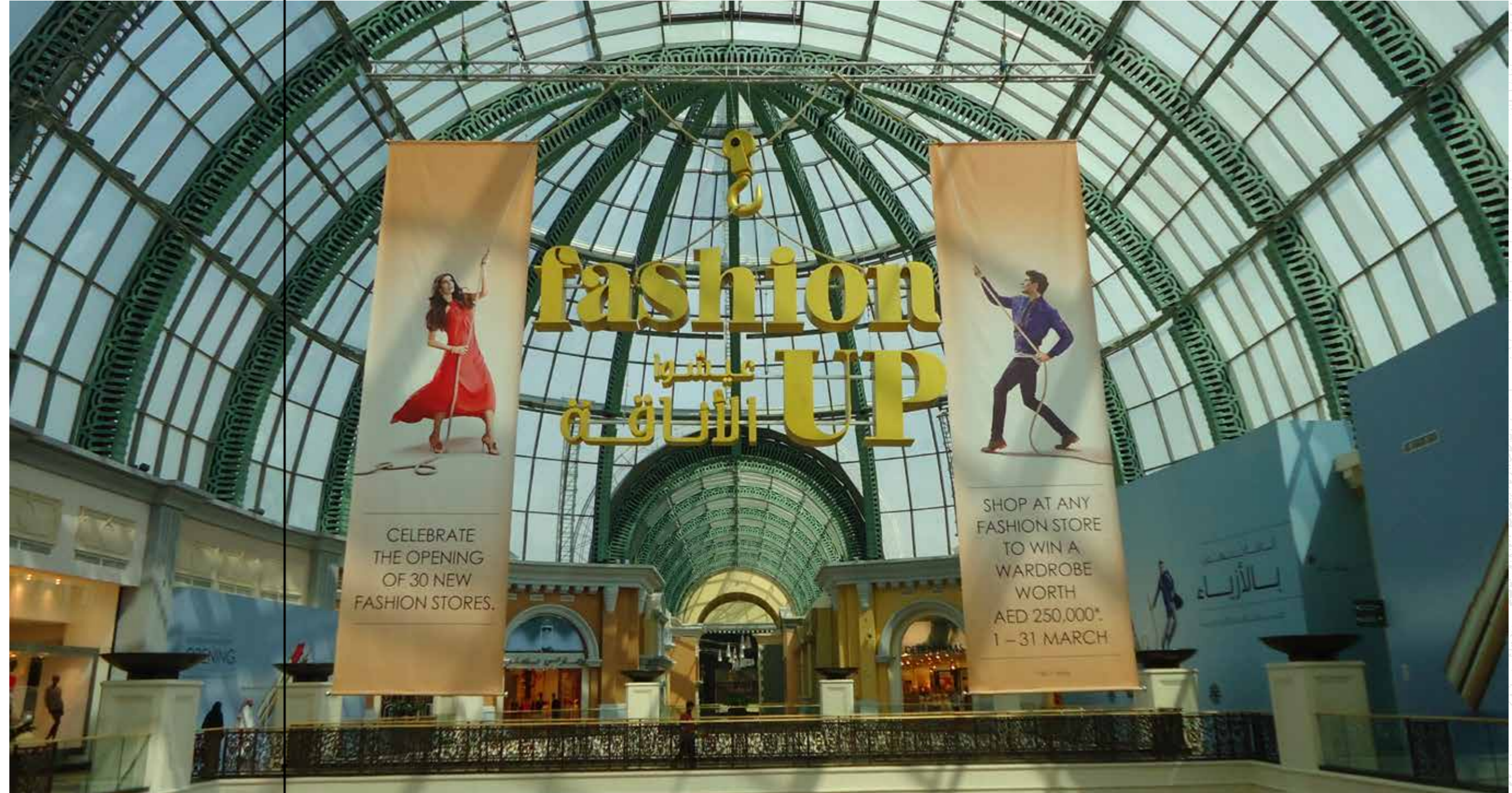
ALUMINIUM TRUSS - CENTER GALLERIA - MALL OF EMIRATES
