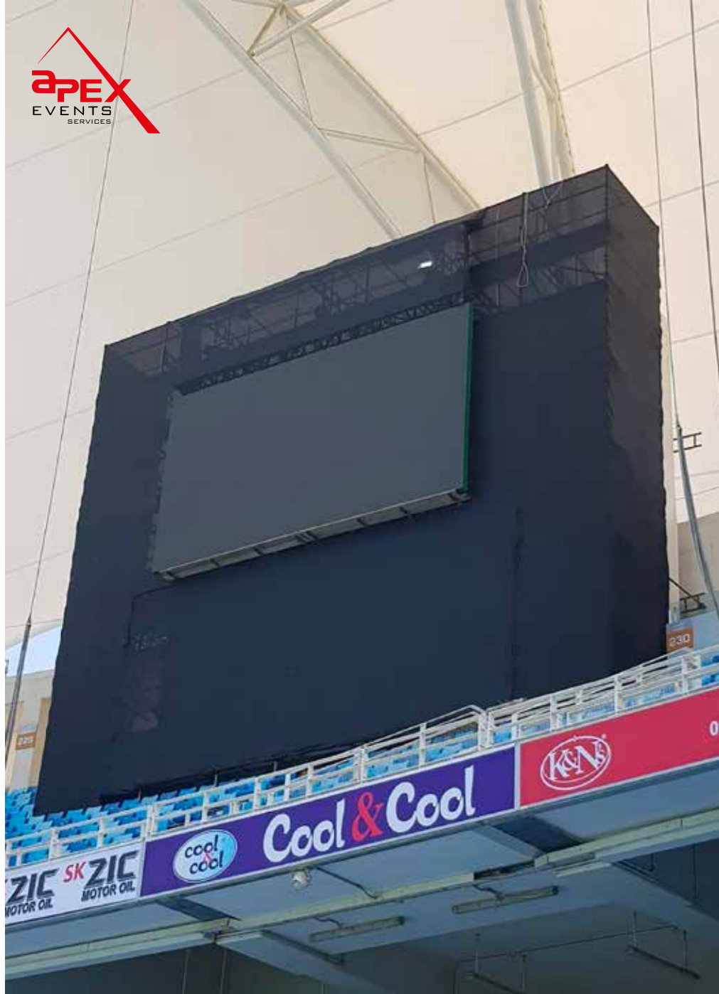
Led Screen Support - Dubai Cricket Stadium
