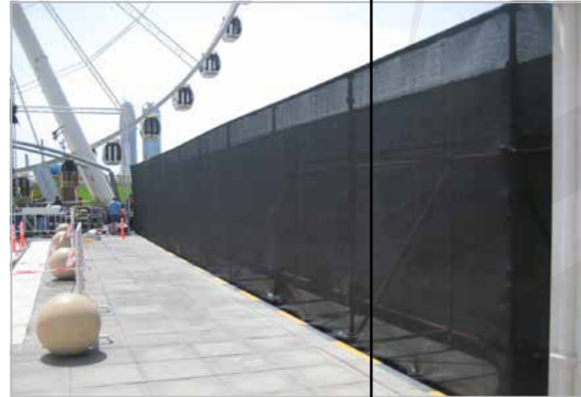
Scaffold Blackout Wall
