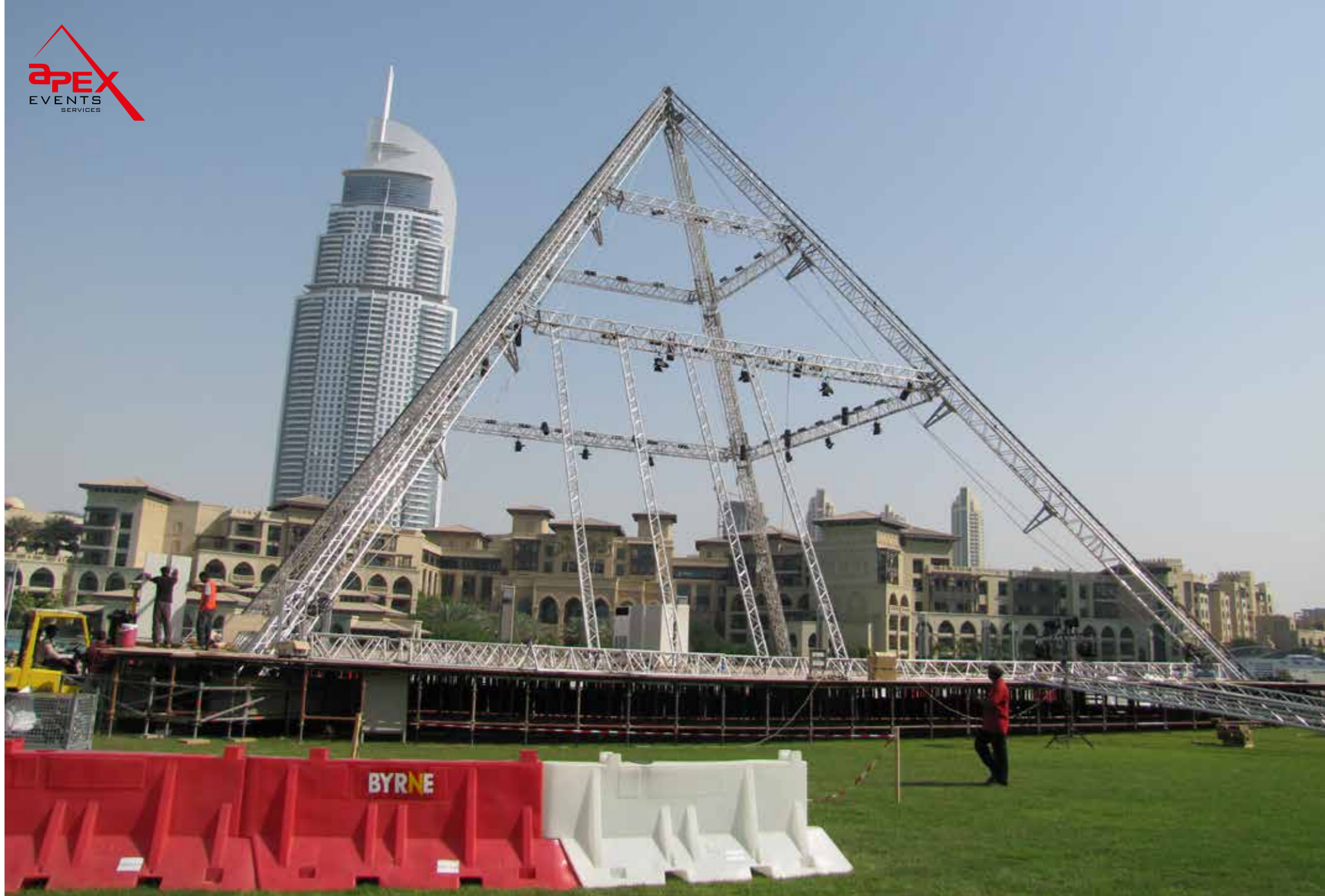
Stage + Triangular Roof Truss - Burj Park - Dubai
