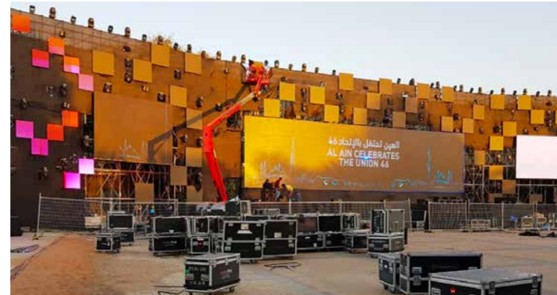
Scaffold Backdrop Structure - 46Th Uae National Day - Al Ain
