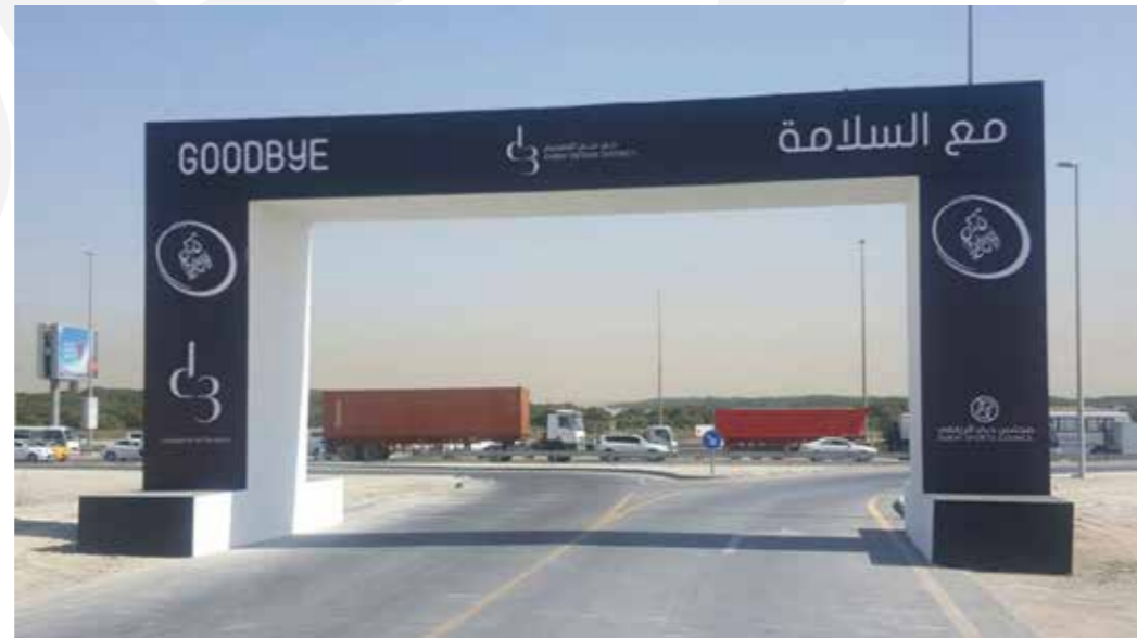
Wide Span Archway Structure - Buisness Bay D3
